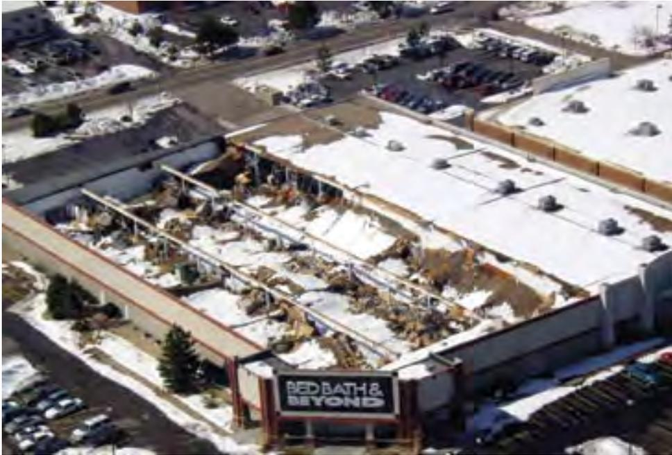
Figure 11. Collapsed roof of the large Bed, Bath, and Beyond store on south College Avenue in Ft. Collins, CO. The roof on this structure was replaced and the store re-opened several months later. Photo courtesy of Ron Phillips, City of Fort Collins.
