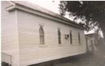
A church in Princeville, NC showing the water marks from the height of the flood (about two-thirds of the way up the windows).
